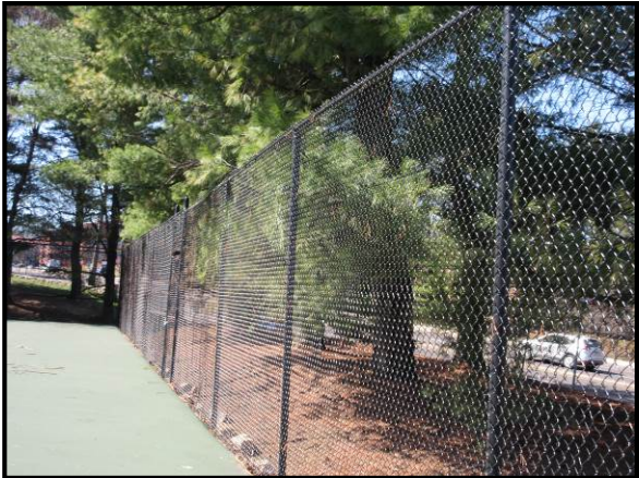
View of chainlink fence at tennis courts
